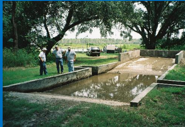
Sand Settling Basin
