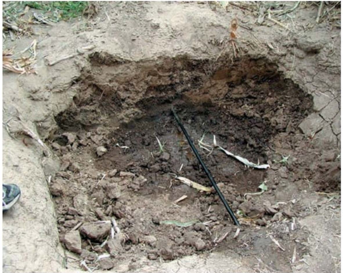
Figure 1. Dripline installed underground.
