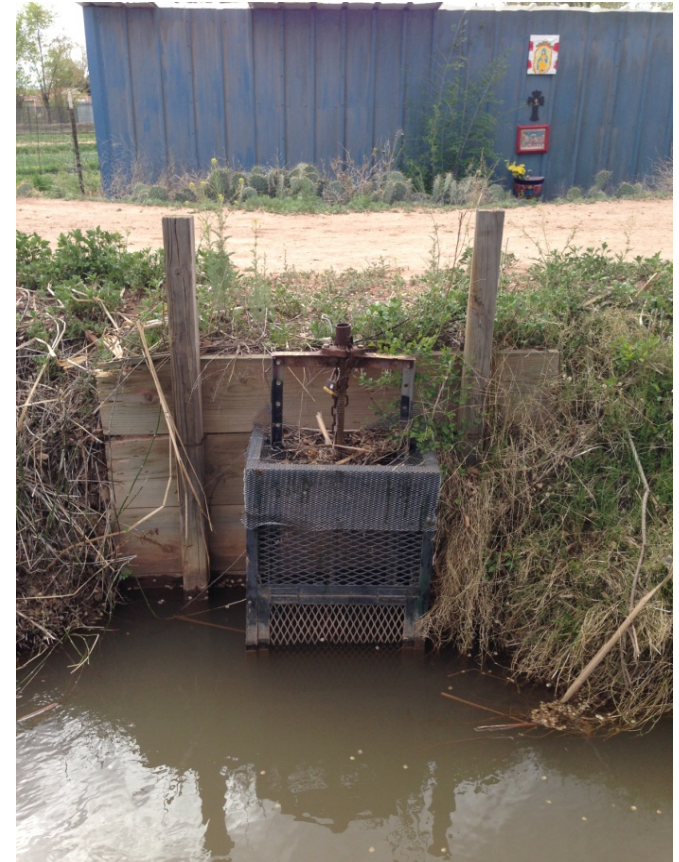
12" turnout into field
