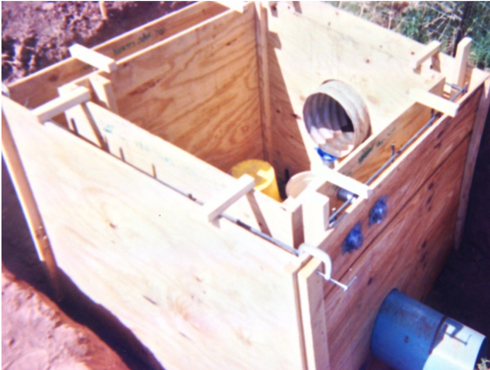
Forming water control structure
