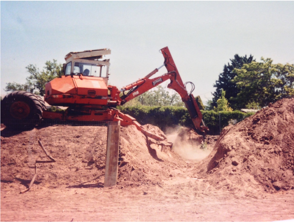
Digging channel for culvert into field
