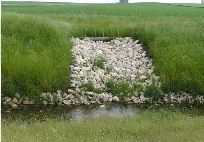
Grade Control Structure in Grassed Waterway
